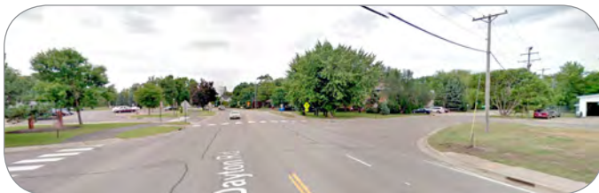
Subsegment B2 intersection of Dayton River Road and Colburn Street - looking northwest, Champlin Source: Google
