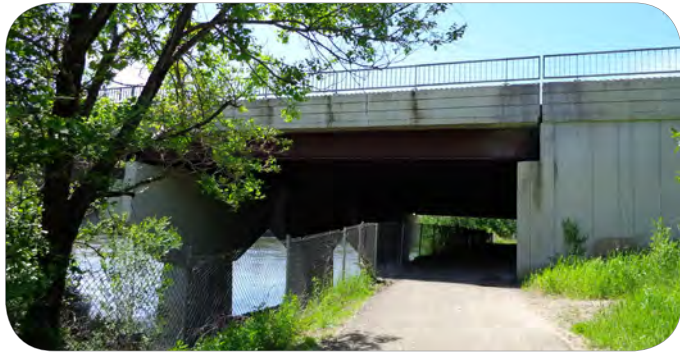
Subsegment D3's I-694 underpass requires attention to improve user experience. Reconstruction plans include new bituminous with improved clear zone, additional tunnel lighting, new fencing, rest stop and wayfinding signage. Source: Three Rivers Park District
