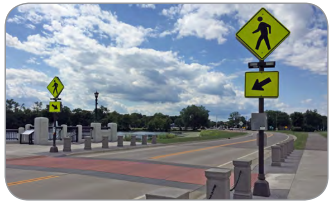
Application of a rapid response flash beacon (RRFB) along WMRR corridor, Champlin. Source: Three Rivers Park District (photo), City of Champlin project
