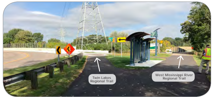
Connection to the Twin Lakes Regional Trail is made here at 57th Avenue N. The WMRRT corridor is seen at right, with the Twin Lakes Regional Trail traversing east. A level A wayfinding kiosk configuration is located at the nexus point of these two regional trails. Source: Three Rivers Park District
