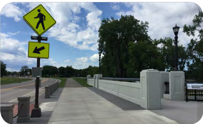
The WMRRT corridor adjacent to the recently reconstructed Elm Creek dam, with the RRFB connection across West River Road.
