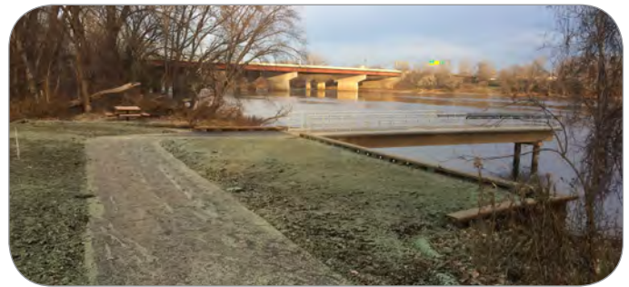
A fishing pier with picnic facilities is located south of the I-694 underpass (I-694 bridge over Mississippi River is noted in background). The retaining wall was recently reconstructed due to ice damage/undermining. Source: Three Rivers Park District
